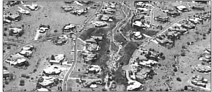
This aerial shot above Elena Gallegos Place clearly highlights the scorched earth around High Desert houses after the May 2018 fire. Seven acres were burned and 10 houses had exterior damage to walls, windows and landscaping. One home had to be entirely vacated and repaired for more than six months due to extensive smoke damage, cracked windows and burned walls.
